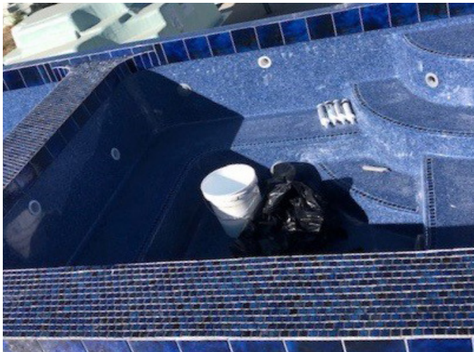
Separator wall covered with ceramic tile.
