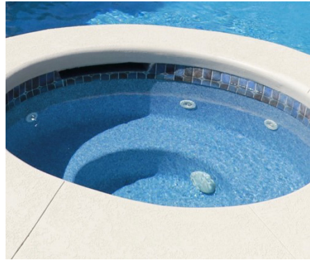
Separator wall covered with cantilever concrete deck.
