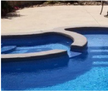
Separator wall covered with cantilever concrete deck. The spillway should be covered as shown per the “Spillways” directives above.
