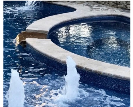
Separator wall covered with pavers and spillway properly covered with stone. Beautiful!
